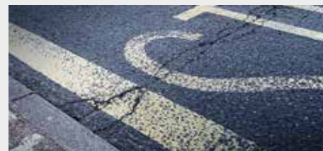
Reflective cracking
