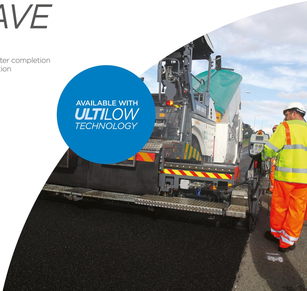
With **ULTIPAVE SINGLE LAYER** both the surface and binder courses can be replaced in a single pass, halving construction time.
