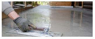
Optimised screed depth and removal of the need to manually mix bagged materials, improves installation time by up to 100%.
